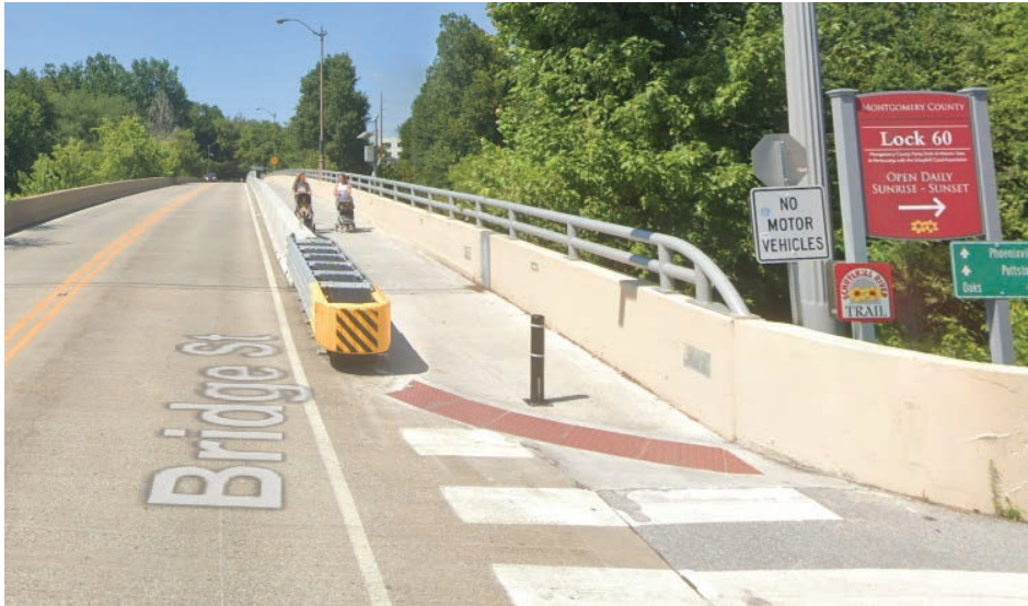
Figure 2.3.08 Example: Retrofitting an existing bridge structure to accommodate a multiuse trail. (Left) BEFORE (2016)-Upper Providence Township, PA. The Schuylkill River Trail over the Schuylkill River. (Right) AFTER (2020)-Upper Providence Township, PA. The Schuylkill River Trail over the Schuylkill River. Note added trail lane width, protection from traffic, rail heights and signage.
