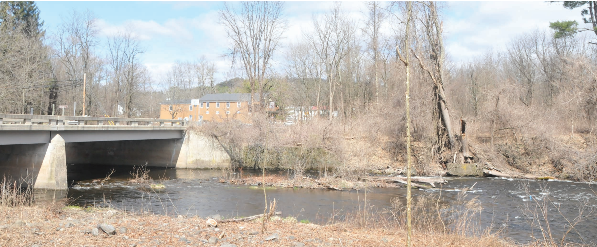
Figure 3.3.03 View to north of the existing Federal 209 Bridge and the highly vulnerable northern stream bank of sedimentary soils directly downstream from the bridge abutment.
