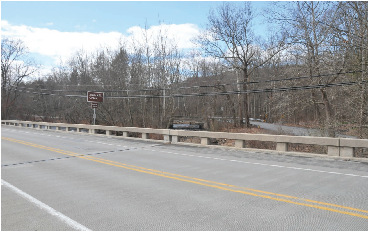
Figure 3.3.02 View upstream across the existing Federal 209 Bridge toward the confluence of the Little Bush Kill with the Bushkill Creek. The southern approach to this bridge is constructed on alluvial materials and is subject to flooding impacts during high flows.
